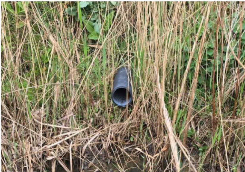
Figure 4 - The pipe is significantly above the water level, even after significant rain in Mid-April.
